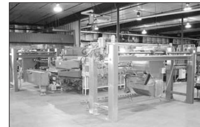
Tempering Line w/ Sanding & Glass Cleaning
