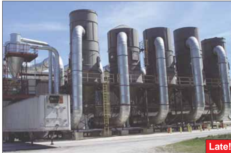
View of Pneumafil (4) 13.5 & (1) 11.5 Dust Collectors
