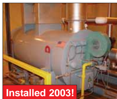
Heatec gas fired boiler
